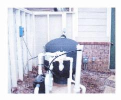
Step 1. Turn-off power to filter pump. Turn multi-port valve to the closed position. Clear work area and observe all safety precautions. For new filter installations, skip to Step 5.
