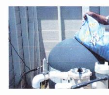
Step 6. Fill filter tank with the required amount of Zeobrite Filter Media. (Note: Zeobrite weighs 50% less than sand per cubic foot, therefore, it requires 50% less weight of Zeobrite versus sand.) See the Media Requireme Chart below.
