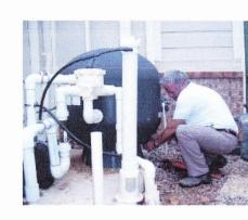
Step 3. If filter is equipped with a drain plug, remove drain plug and drain wate from filter tank.
