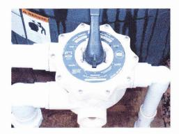
Step 8. Turn multi-port valve to the backwash position. Start filter pump and backwash the media until the water in the site glass is clear (usually 2-3 minutes). Turn-off filter pump and proceed to Step 9
