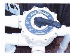
Step 9. After backwash, move multi-port valve to the rinse position and run until water clears in the site glass. Turn-off filter pump, move multi-port valve to the closed position and proceed to Step 10.
