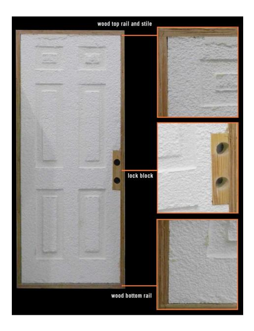
This example below provides composite bottom rail while the stiles and top rail is entirely made of wood. The composite bottom rail stops the moist from entering but allows water to penetrate from the stiles which will cause damage to the door. Most of the strength comes from the polyurethane foam that is injected into the door. Air holes present inside the door leads to less durability.
