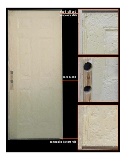
This last example of fiberglass door illustrates one that is made of wood rails and stiles all around the door. The door is a combination of steel wood and foam. The all around wood rails and stiles allow water and moist to enter and damage the door similar to the other doors mentioned above..
